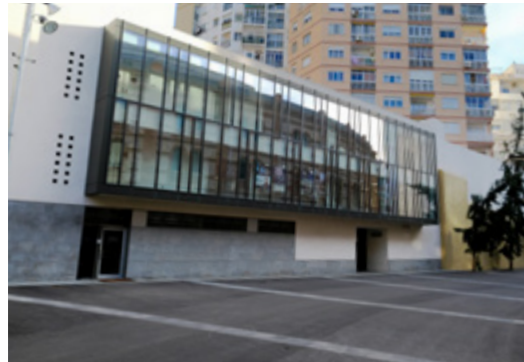
2 Backstage i aparcament privat. Backstage i aparcamiento privado. Backstage and private parking.
